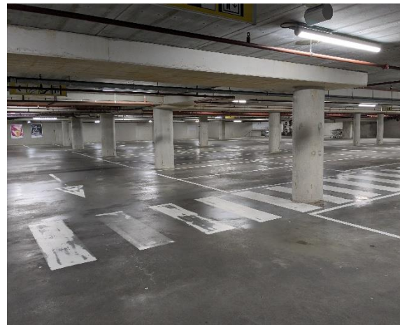
Figure 3 Parking garage less than 200m away from Kavel 5 (own picture)
